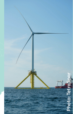
TetraSpar Demonstrator (Norway) COD 2021: working in partnership with Stiesdal Offshore Technologies, Shell and TEPCO to deploy a tubular steel structure with a suspended keel
