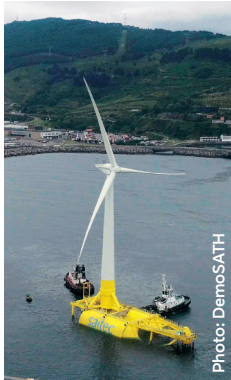
DemoSATH (Spain) COD 2023: working with Saitec to deploy a concrete twin-hull barge structure with a single point of mooring
